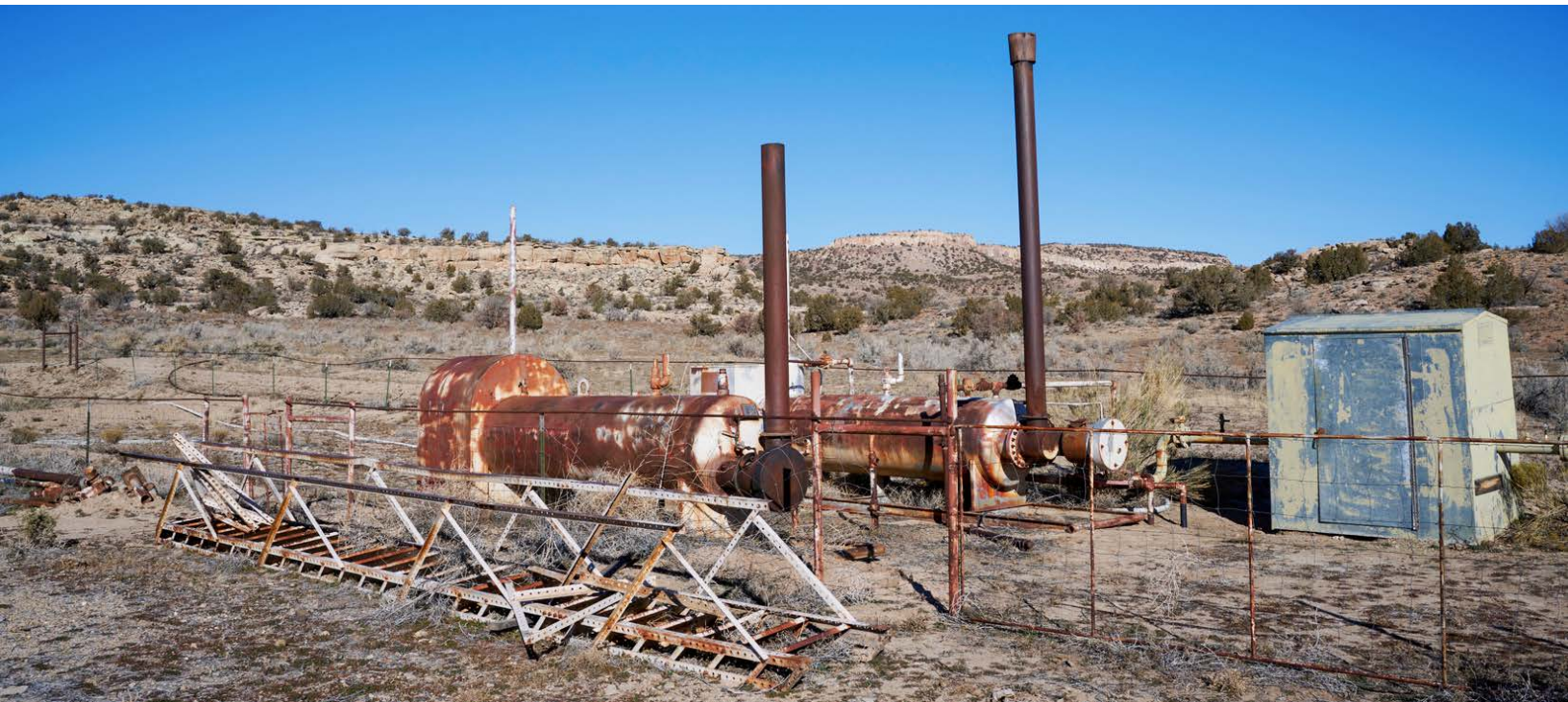
Above: Abandoned oil and gas infrastructure on federal public lands near Hovenweep National Monument. PHOTO: JON MULLEN Above right: Pueblo site in Montezuma Canyon, Southeast Utah. PHOTO: PAUL REED
