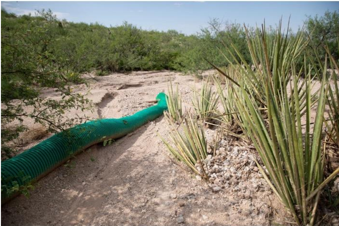
Figure 4. Silt fences made of synthetic material dispersing into the drainages near 32.364137°, -110.492155°, July 29, 2024.
