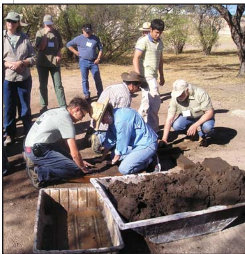
Left: Participants get their hands dirty making adobe bricks. Right: Boiling alum, which is then applied to lime plaster as a traditional waterproofing technique.
