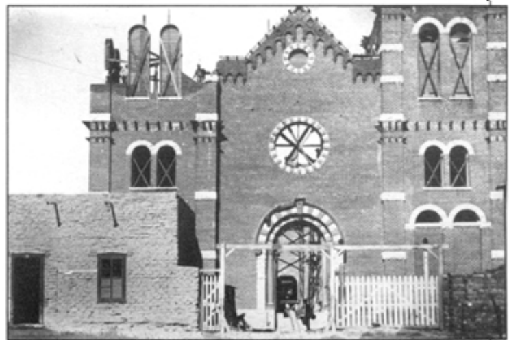
The St. Augustine Cathedral on Stone Avenue under construction in 1896. Quintus Monier built it in part with bricks manufactured at his brickyard on West Congress Street (later the Tucson Pressed Brick Company). The adobe building in the foreground is typical of structures replaced as local brick production increased (photo no. B.92, 788-92, 791 courtesy of the Arizona Historical Society).
