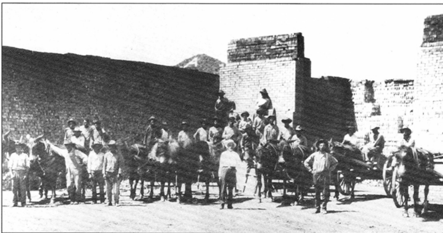
Employees of the Tucson Pressed Brick Company posing in front of a partially constructed scove kiln (photo no. B92,788-92,791 courtesy of the Arizona Historical Society).
