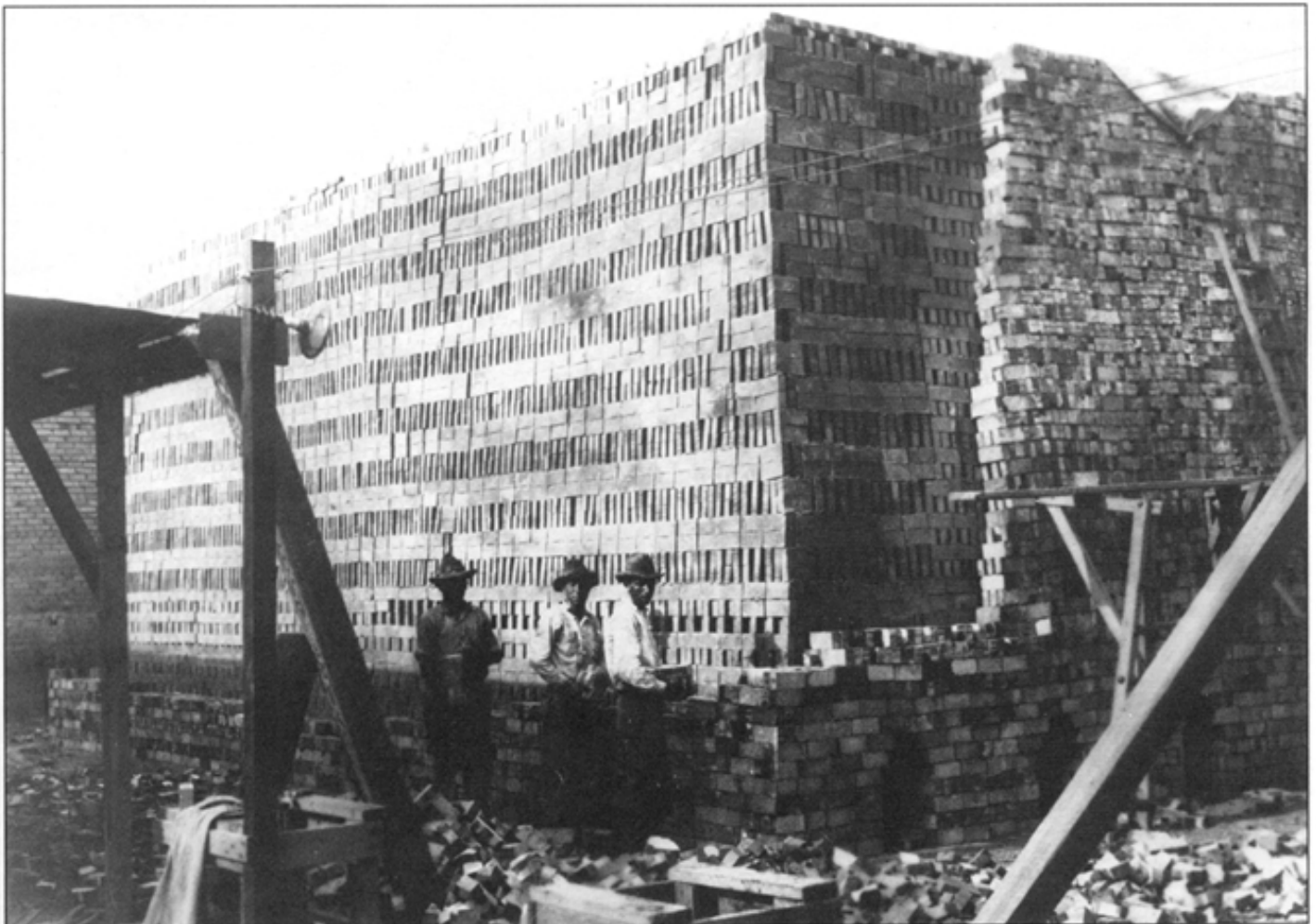
Laborers constructing a rectangular scove kiln. Coal was placed into the horizontal flues visible in the lower right portion of the photograph and set afire (photo no. B.92,788-92,791 courtesy of the Arizona Historical Society).
