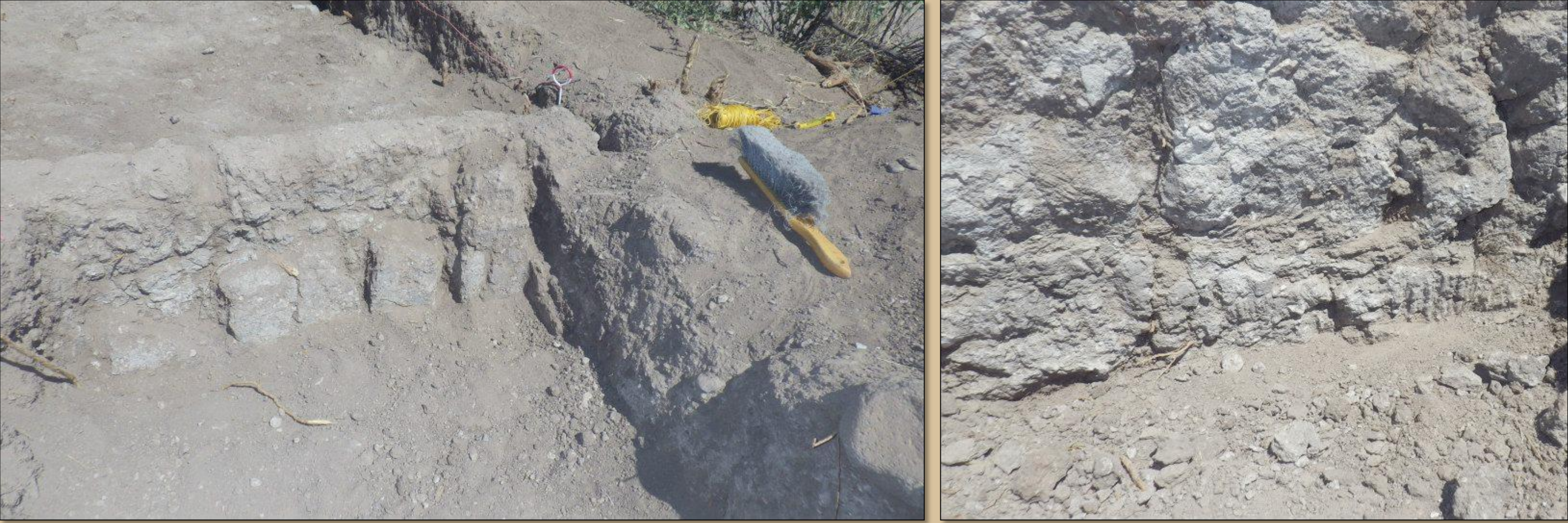
Above: Left: Photo of adobe buttress stabilizing an interior wall; Right: Photo of reed impressions in adobe wall.
