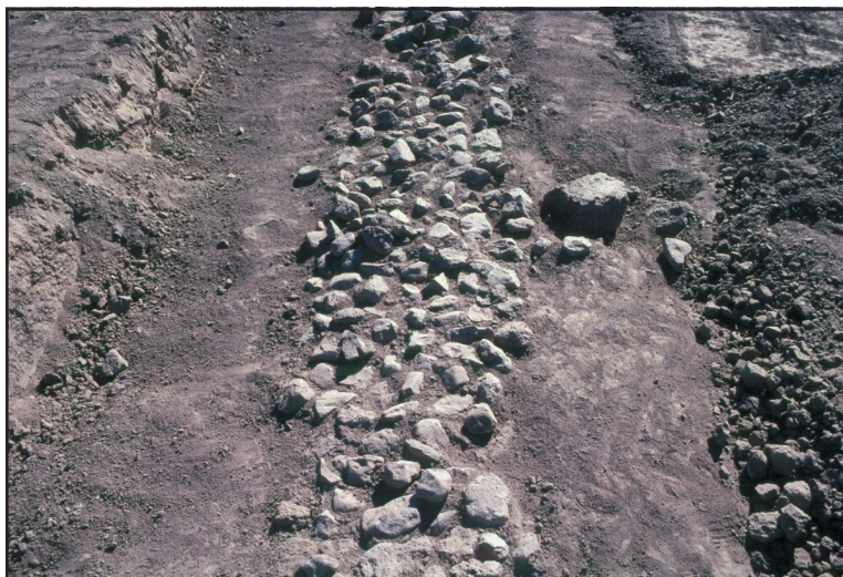
Figure 4.28. Feature 3026, the foundations of the eastern gardens wall, Mission Gardens locus, the Clearwater site, AZ BB:13:6 (ASM).
