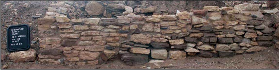
Example of Wall Type 7, from Room 118.
