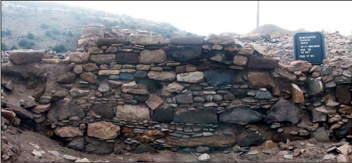
Example of Wall Type 13, from Room 76.
