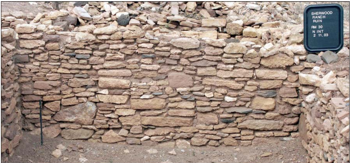
Figure 4: Stone wall from Southern Pueblo utilizing tabular sandstone. Western Mapping wall type # 2 (see Appendix 1)
