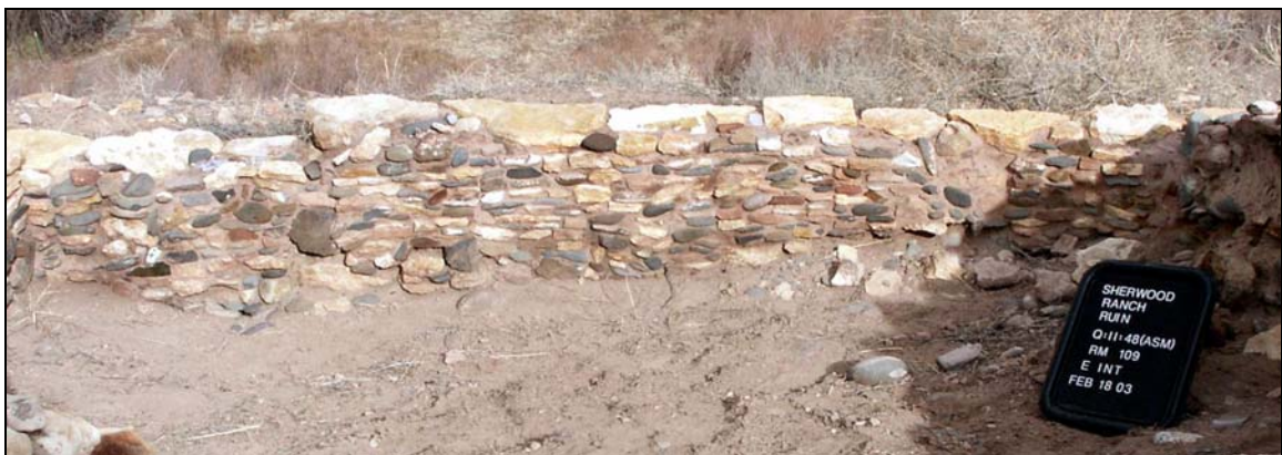
Example of Wall Type 16, from Room 109.
