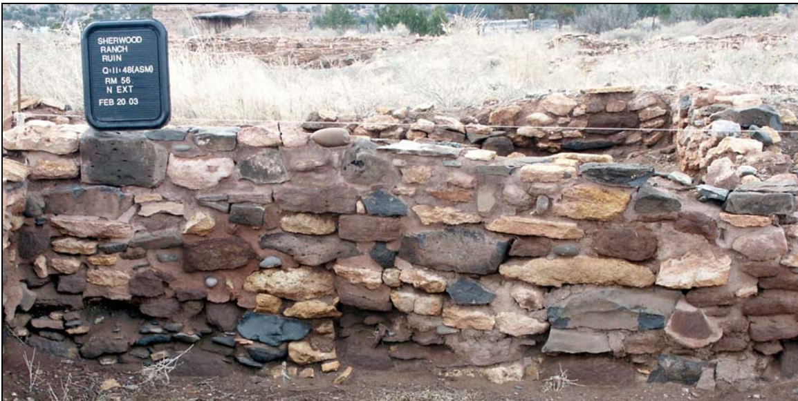
Example of Wall Type 10, from Room 56.
