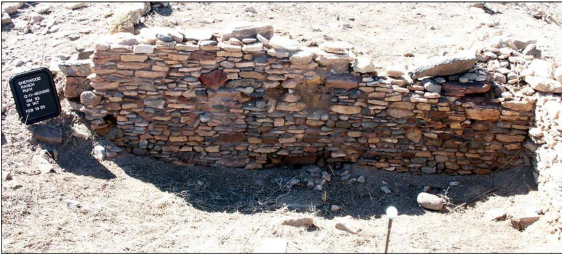
Figure 2. Typical masonry wall in Northern Pueblo, utilizing mixed types of stone.
