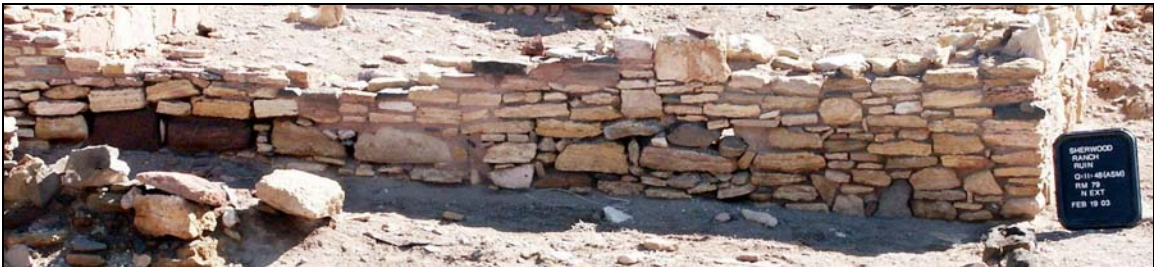
Example of Wall Type 14, from Room 79.
