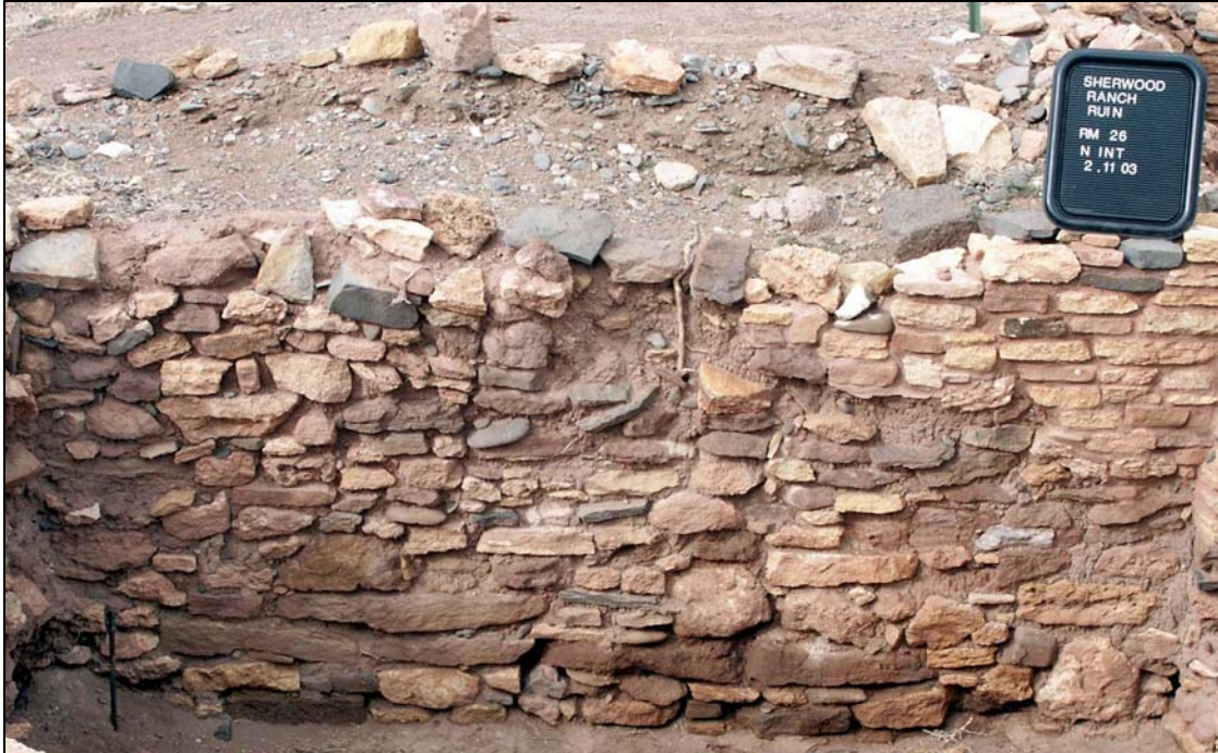
Example of Wall Type 1 from Room 26.
