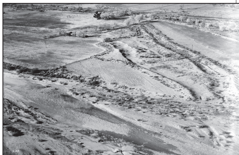
Top: Mosaic photograph of Tempe and Mesa, showing canals with Halseth's annotations, January 1930. Historic canals were identified with red ink; prehistoric canals were marked in green. Bottom: Oblique aerial photograph of prehistoric canals at Pueblo Grande, Park of Four Waters, looking northwest, January 1930. (Both photographs courtesy of the National Anthropological Archives, Smithsonian Institution, Photo Lot 3, and Pueblo Grande Museum, City of Phoenix.)
