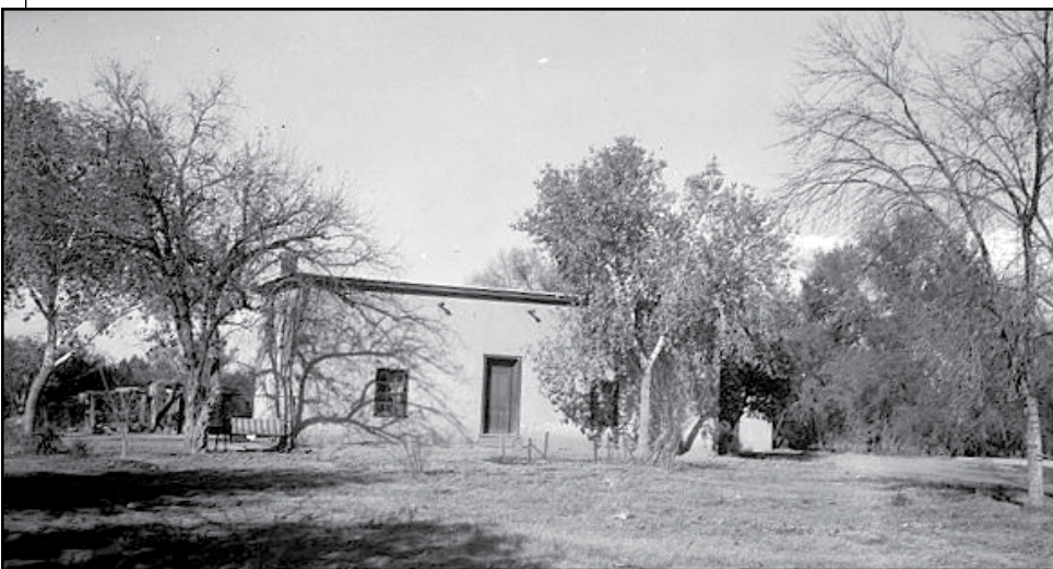
León family house, 1937 (photograph by Frederick A. Eastman, Historic American Buildings Survey collection).
