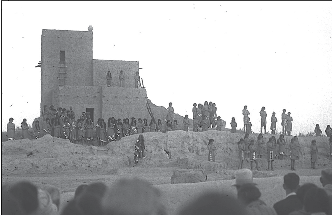
For the pageants held at Casa Grande Ruins National Monument from 1926 to 1930, a stage and multistory “adobe,” made of wood, were constructed in Compound B, 500 yards from the main ruin. This photograph was taken in November 1926 by Edwin F. Carpenter, a young astronomy professor at the University of Arizona.
