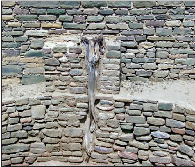
Juniper was used most extensively by Salmon Pueblo's inhabitants during the second occupation. This room contains a large juniper post embedded into a kiva pilaster.
