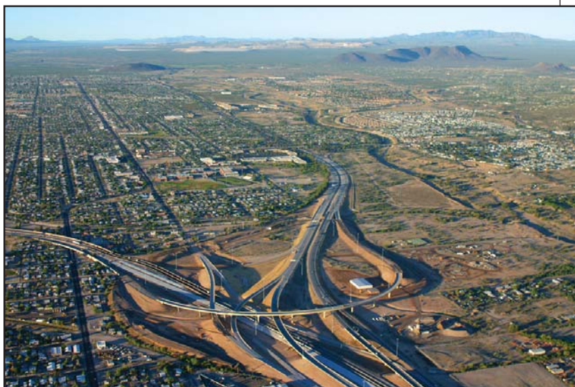
The large scale of the interchange for Interstate 10 and Interstate 19 created open space that could be used as an archaeological preserve, which was expanded further with transportation enhancement grant funds.
