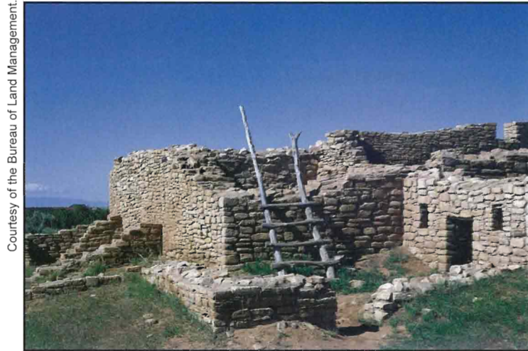
Lowry Pueblo National Historic Landmark.
